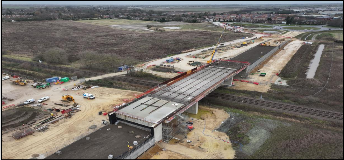
SWRR – Reinforced Concrete Deck Pours
