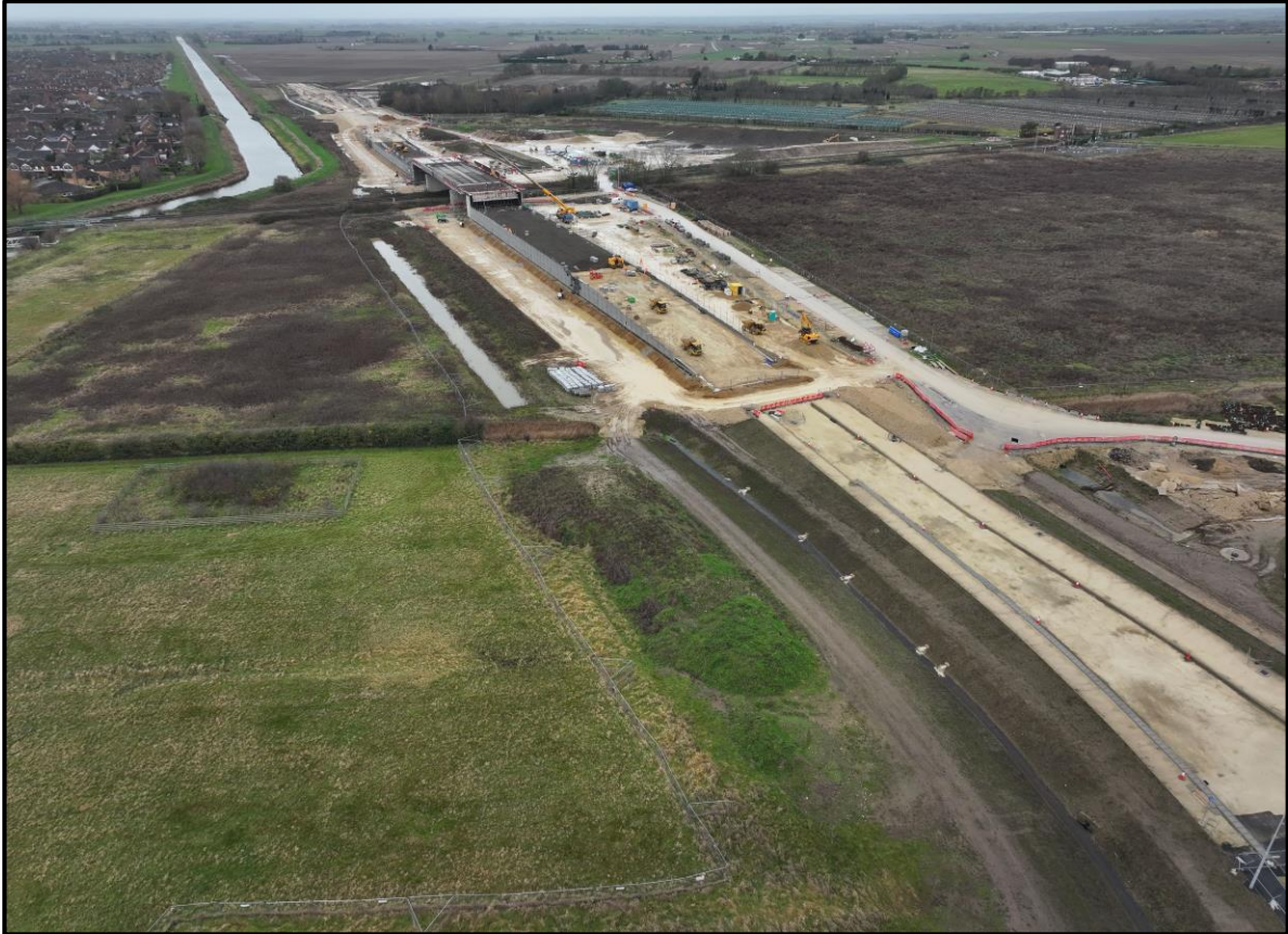
SWRR – Aerial view from Enterprise Way Looking West along Vernatt’s Drain
