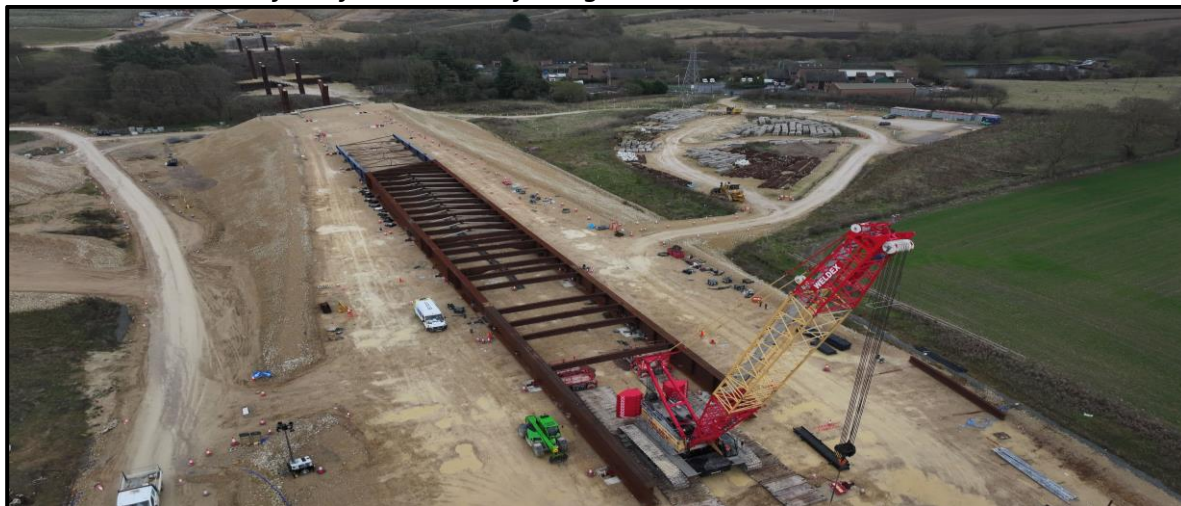
GSRR – Fabrication of the first section of bridge between west abutment and Pier 1
